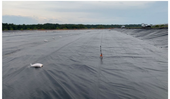
Example of prepared dewatering pad utilizing 24 mil Woven Coated PE Liner
