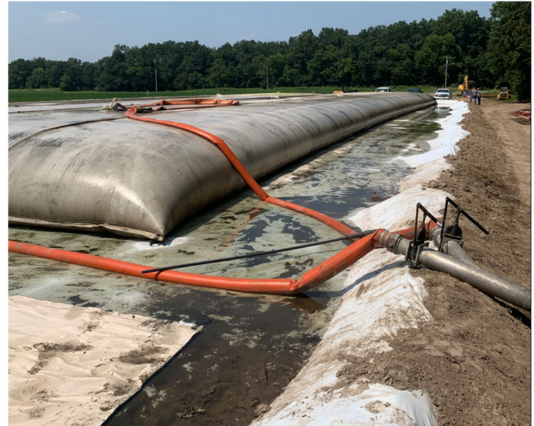
Example of mechanical valves to control rate of discharge to the Geotextile Tube
